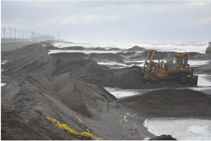
Figure C.1.6 - A 5 mile gravel berm provides insufficient shoreline protection from coastal erosion in Utqiagvik and must be repaired after every storm, as shown above, which costs $8.3 million annually. A $328 million U.S. Army Corps of Engineers project will construct a fortified rock revetment to protect the shoreline and requires the North Slope Borough to contribute $110 million due to USACE non-federal cost share requirements. Virtually no other rural Alaska community has the resources to complete a similar project. Credit: North Slope Borough.
