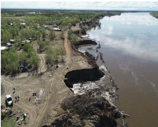
Figure C.1.5 - In 2018, sections of the riverbank in Huslia were lost to rapid erosion, shown above. Erosion is expected to impact water and sanitation infrastructure in summer 2020, resulting in approximately $2 million in damage and loss of service to 70 homes. Traditional water and sanitation funding sources do not fund the modifications that Huslia needs to preserve water service to homes. The community is uncertain where funding will come from. Credit: Huslia Village; 2018.
