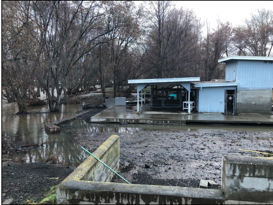
Figure C.2.6 - “The lamprey restoration project on the Confederated Tribes of the Umatilla Reservation, near Mission, Oregon, was completely destroyed by recent flooding. Tanks full of some 1,500 eels washed away. The tribes are working to restore this valuable traditional food source by rearing juvenile lamprey” Source: King, A. Northwest News Network (Davis, 2020).
