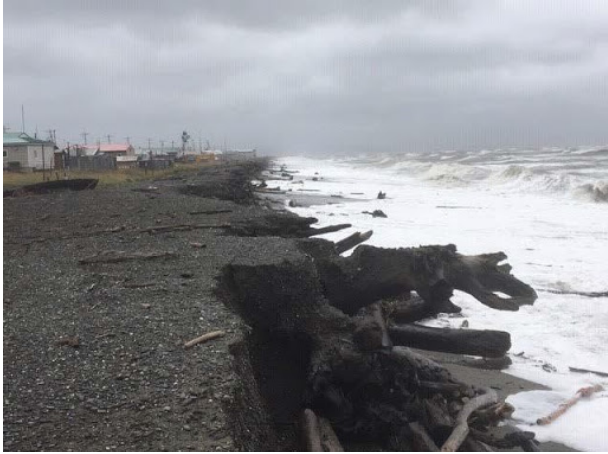
Figure C.1.2 - On August 2, 2019, an unusual summer storm washed 350,000 cubic feet of Shaktoolik's storm surge berm into the Bering Sea, leaving all of the community's infrastructure highly vulnerable to fall storms (shown above). More funding is needed to complete berm construction, which will likely serve as a temporary solution--until funding for a rock revetment can be secured or relocation to a safe site 14 miles away is determined to be the only long-term solution. Credit: Katchatag, Sophia; Native Village of Shaktoolik; 2019.
