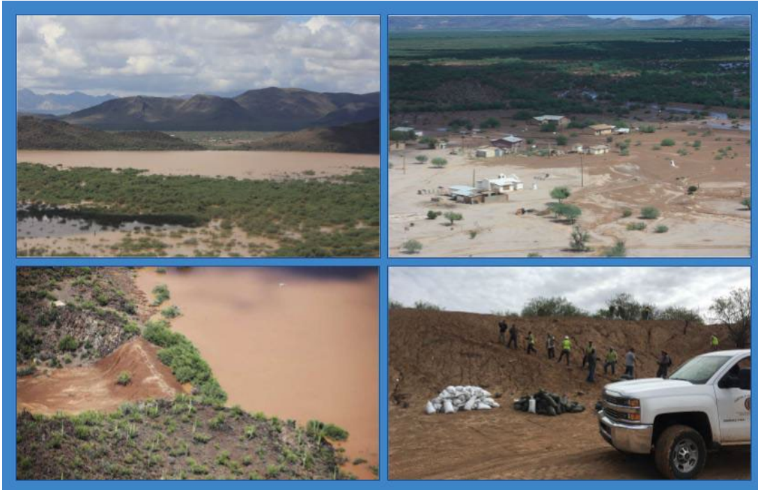
Figure C.2.9 - Upper left: “Meneger’s Dam Lake. At the center of the image is the earthen embankment of the dam; just beyond the embankment the community of Meneger’s Dam can be seen”. Lower left: “The earthen Menagers Dam is in imminent danger of failing, potentially sending floodwaters rushing into the Tohono O’odham Village of Ali Chuk . . . after Hurricane Rosa’s remnants drenched the western half of Arizona”. Upper right: “Kohakt Village, the saturation in the ground indicating where water had flooded” Lower right: “Sandbagging operation to shore up the berm at Meneger’s Dam”. Photo credits: Richard Saunders, Tohono O’odham Nation Director of Public Safety. (Tohono O’odham Nation, Office of the Chairman and Vice Chairman, 2018c); Lower left: Mike Christy/Arizona Daily Star via AP (Anonymous] New Haven Register 2018 October 5 ‘Southern Arizona dam holding as water recedes’).
