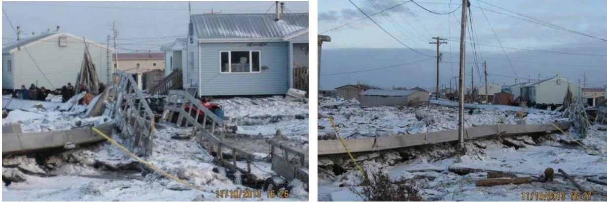
Figure C.1.9 - In November 2013, an ice-jam flood inundated the entire community of Kotlik, resulting in a federal disaster declaration and causing $9.8 million in damages to the water and sanitation system alone. Although Kotlik received funding to rebuild after the disaster, the community has struggled to secure funding to take proactive action to protect community infrastructure before erosion causes a disaster in their community. Kotlik needs to develop a new subdivision site to relocate at least 21 homes threatened by erosion. Credit: Village of Kotlik; 2013.
