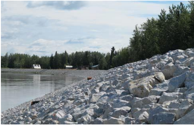
Figure C.1.4 - In 2010, McGrath armored their riverbank to protect infrastructure from erosion with assistance from the Natural Resources Conservation Service Emergency Watershed Protection program, which has been effective in helping Alaska Native villages address climate impacts to infrastructure. Photo Credit: Natural Resources Conservation Service; 2015.
