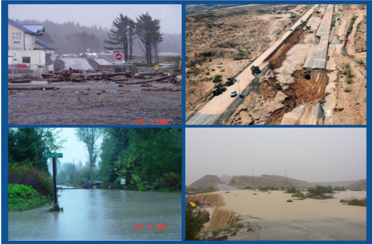
Left side: The Quileute Tribe has endeavored to relocate over the past decade in response to the impacts of storm surges amplified by sea level rise. Climate impacts have severely damaged the Tribe's infrastructure, including transportation, residences, and centers for education and business. Washington State. Image credit: Quileute Tribe Hazard Mitigation Plan, 2015. Right side: Severe flooding has repeatedly impacted the Moapa Band of Paiute Indians reservation, including the adjacent I-15. The Tribe still had not received its federal funding 13 months after the flood. Image credits: Moapa Band of Paiutes Hazard Mitigation Plan, 2015.
