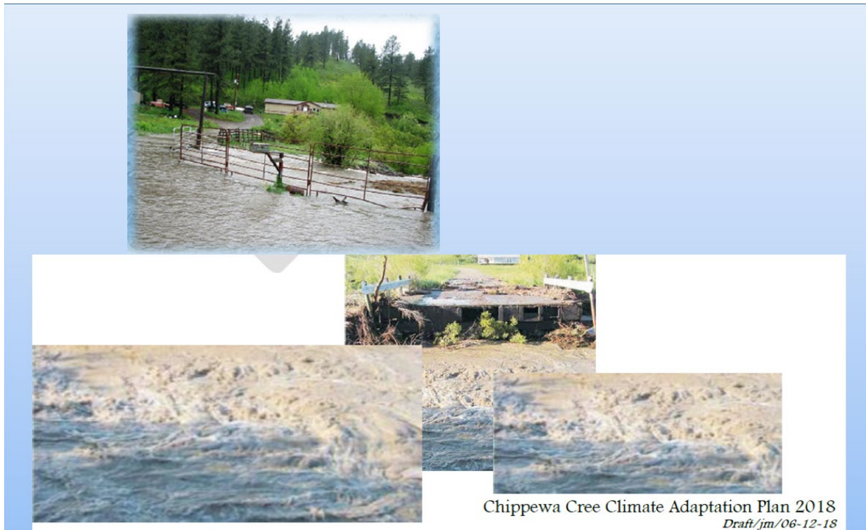
Figure B4.3 - Impacts of severe precipitation events on transportation infrastructure, Chippewa Cree community (Chippewa Cree Climate Adaptation Plan, 2018.)
