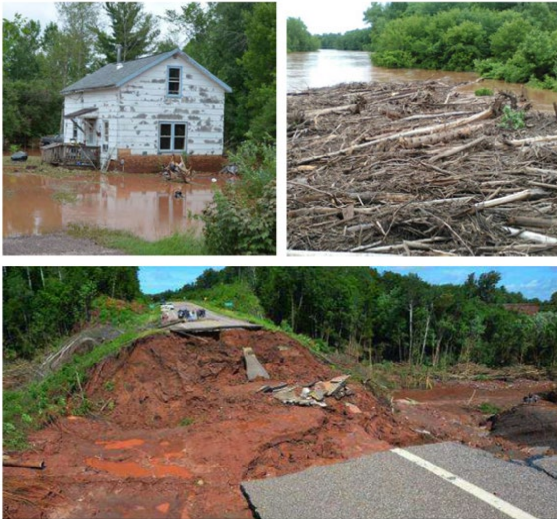
Figure B6.3. Flood impacts on Bad River Reservation infrastructure, July, 2016. (Source: Kilger and Brock-Montgomery, 2018).
