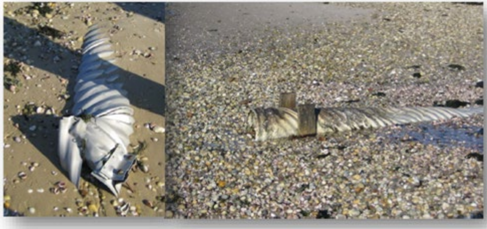
Figure C.2.10 - Culverts, pipes adjacent to Shinnecock Indian Cemetery. Pipes are clogged, and in need of repair.
