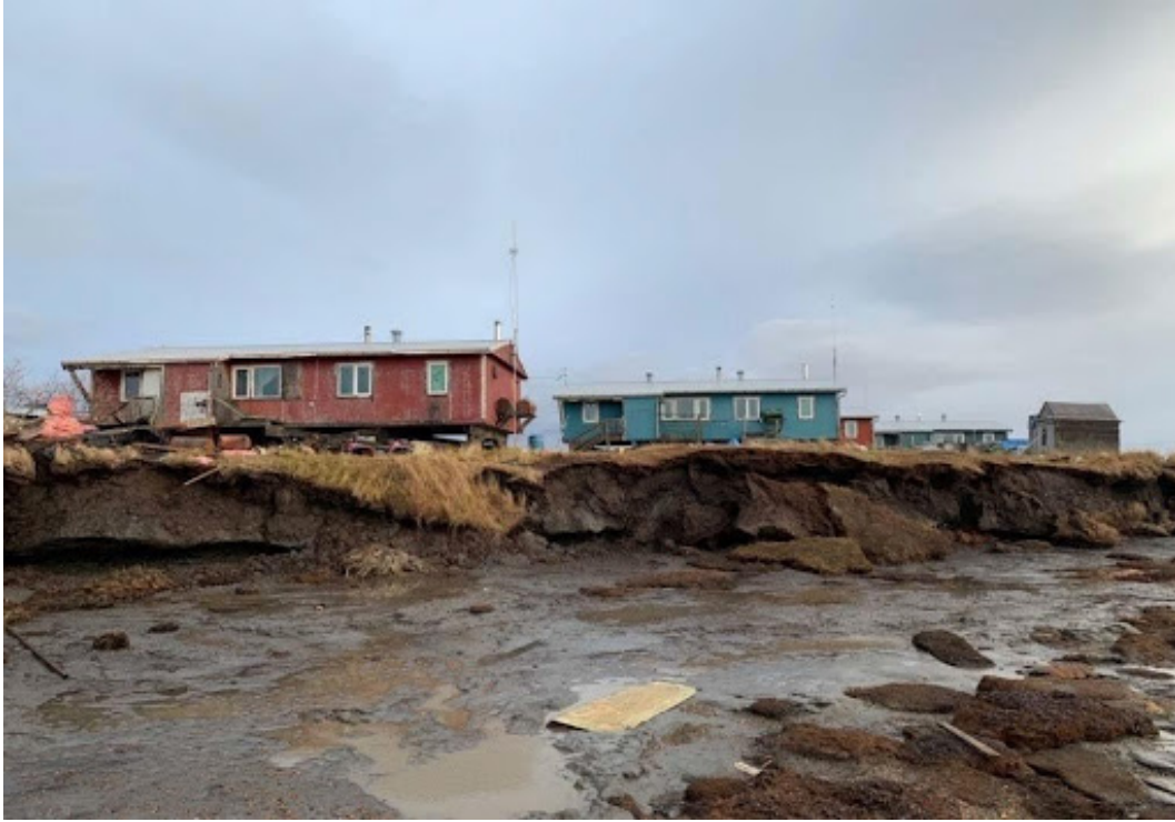
Figure C.1.7 - The eroding riverbank (shown above in 2018) forced Newtok to demolish the homes shown above in 2019 to prevent collapse into the river. For communities like Newtok, taking proactive action to respond to climate impacts would result in millions of dollars in savings as compared to responding to disasters. Credit: John, Andrew; Village of Newtok; 2018.
