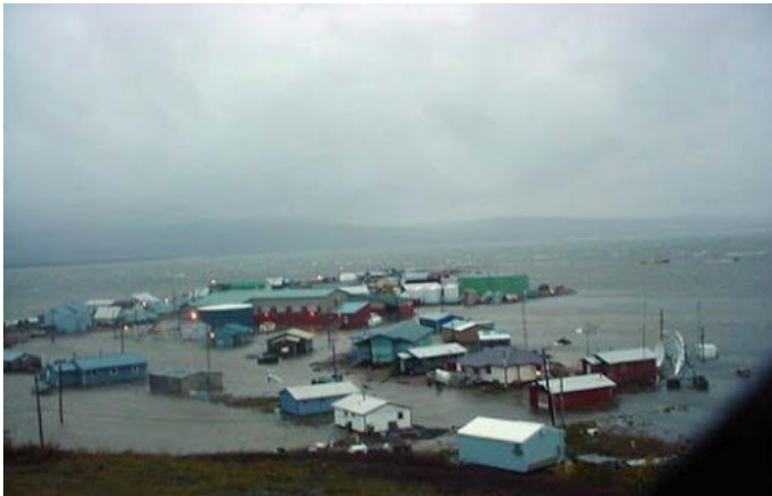
Figure C.1.11 - In September 2005, a severe fall storm caused flooding of the entire spit in Golovin, where the school, power plant, fuel tank farm, clinic, and other critical infrastructure are located. In order to protect from flooding, Golovin is planning to migrate all community infrastructure from the spit to an area of higher ground adjacent to the community, an immensely complex process. Small communities such as Golovin benefit from technical assistance to complete large-scale projects such as managed retreat. Credit: Chinik Eskimo Community; 2005.
