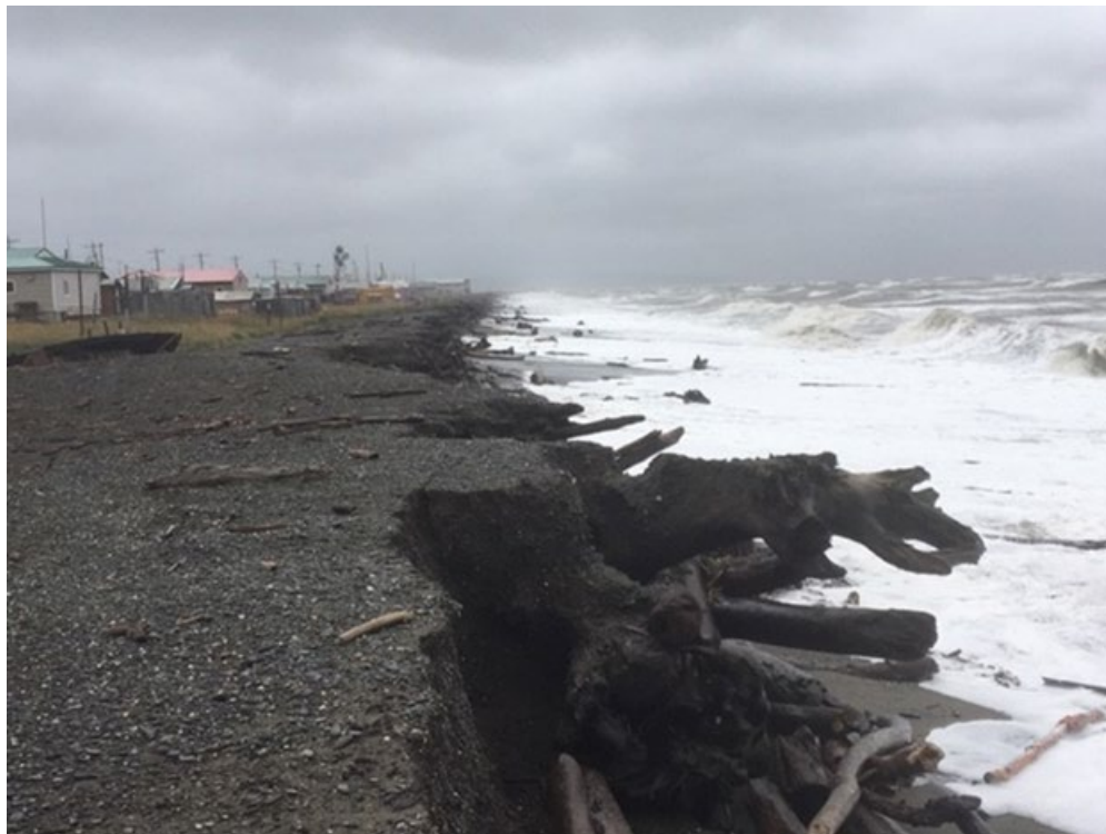
Figure 5. On August 2, 2019, an unusual summer storm washed 350,000 cubic feet of Shaktoolik's storm surge berm into the Bering Sea, leaving all of the community's infrastructure highly vulnerable to fall storms (shown above). Shaktoolik must apply to a myriad grant programs across many different state and federal agencies to secure funding to respond to their threat. Credit: Sophia Katchatag, Native Village of Shaktoolik.
