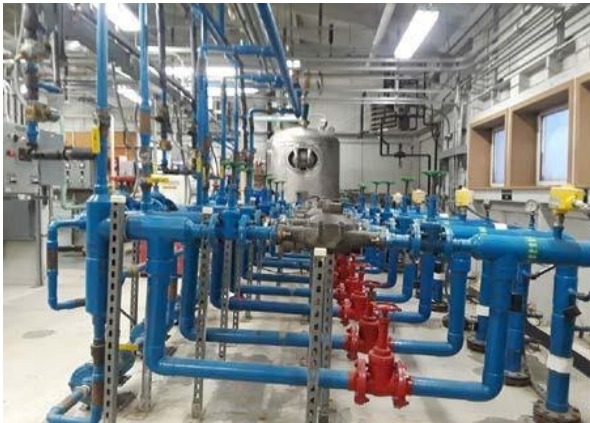
Figure C.1.8 - Thawing permafrost in Noatak is causing infrastructure to fail. Paul, the water and sewer operator, is constantly repairing leaking pipes due to the settling ground. For example, ice settling last summer – the hottest on record – broke a pipe and it took a month of digging and investigation to find the leak. The increasing damage from permafrost thaw is a sign that significant adaptation solutions must be implemented soon in order for the community to continue to have running water and flush toilets. Credit: Alaska Native Tribal Health Consortium.
