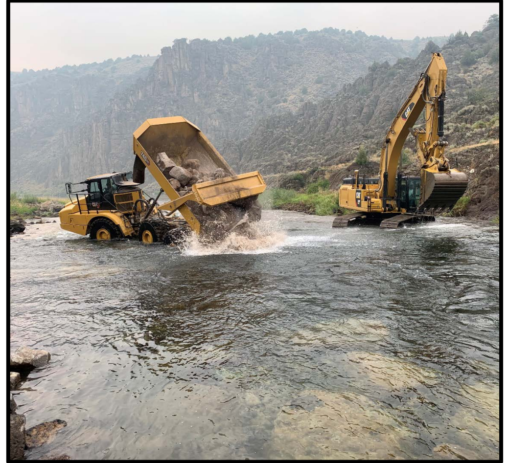
Photo: Reclamation constructing a new riffle in the Teton River downstream of remnants of Linderman Dam (Idaho) to improve habitat, resolve a public safety issue and provide reliable irrigation, October 2021.
