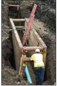
Workers utilize a trench box to guard against cave-ins during their water and sewer pipe installation.
