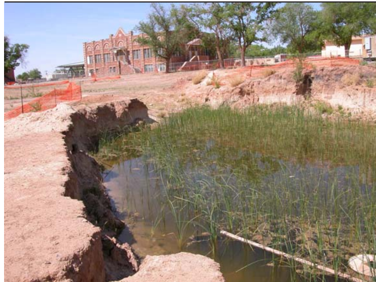
An excavation at Tuba City Boarding School reveals shallow groundwater.
