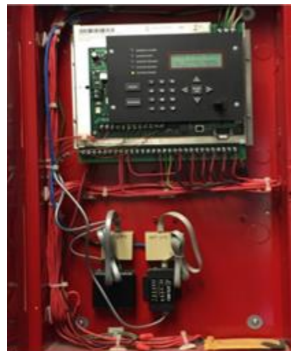
Automatic Sprinkler System Panel
