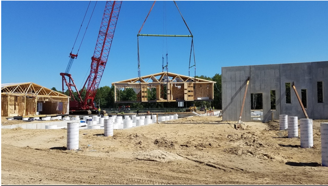
Placing a Module On-Site for the Construction of the Bug-O-Nay-Ge-Shig High School in MN
